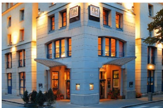
NH Salzburg City 140 rooms
